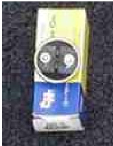
ITEM 5-Pressure switch for turning on fans
